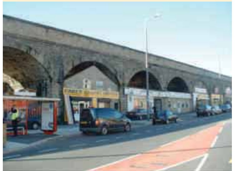
Stanningley Railway Viaduct
